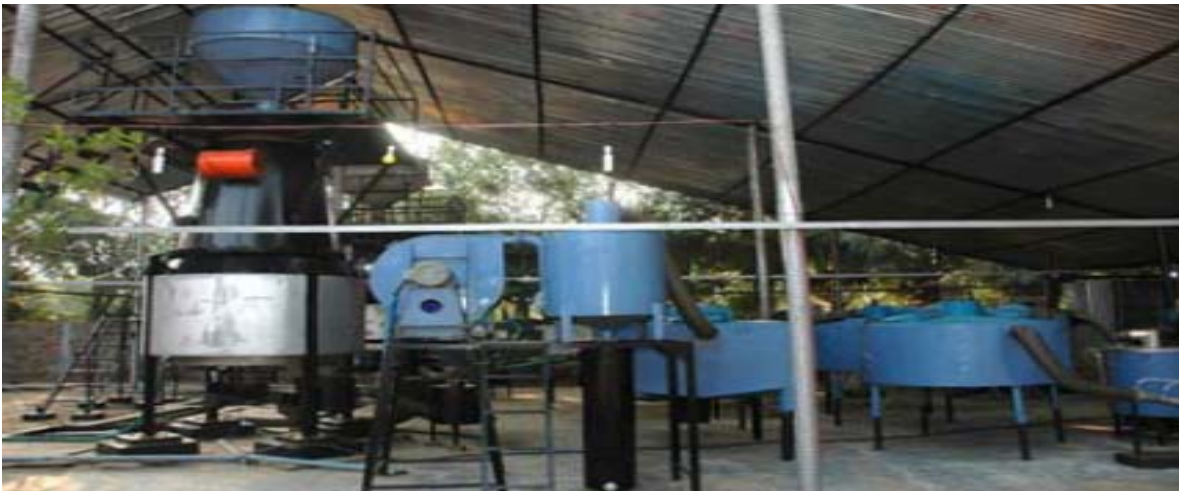
Figure 1: Front face of power plant
