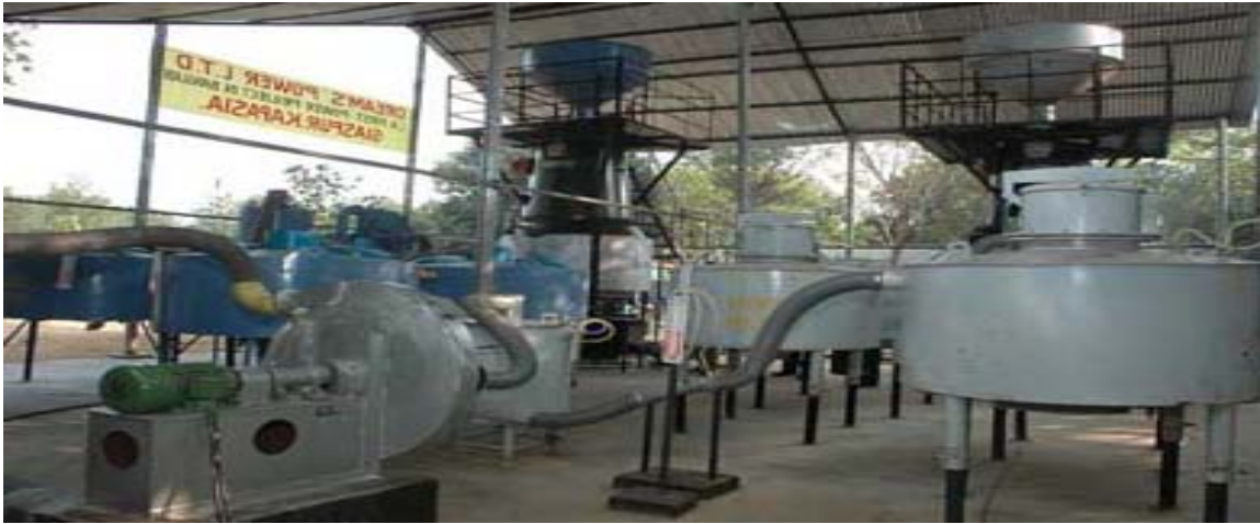
Figure 2: Gasifier Unit of the power plant
